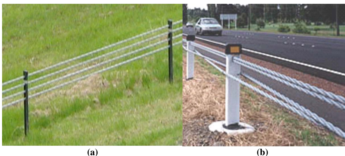
Figure 1 – photos of two forms of wire rope barrier, (a) four-rope parallel and (b) two parallel, two intertwined. Sources: Candappa (a); and Larsson et. al. (2003)
