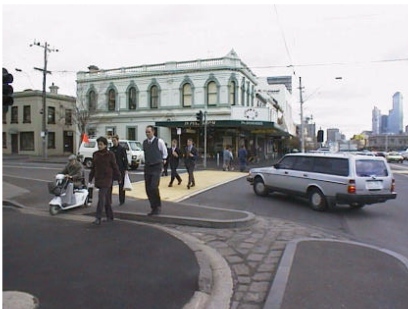
Figure 2.4: Pram crossing installed on existing pedestrian crossings at Clarendon Street
