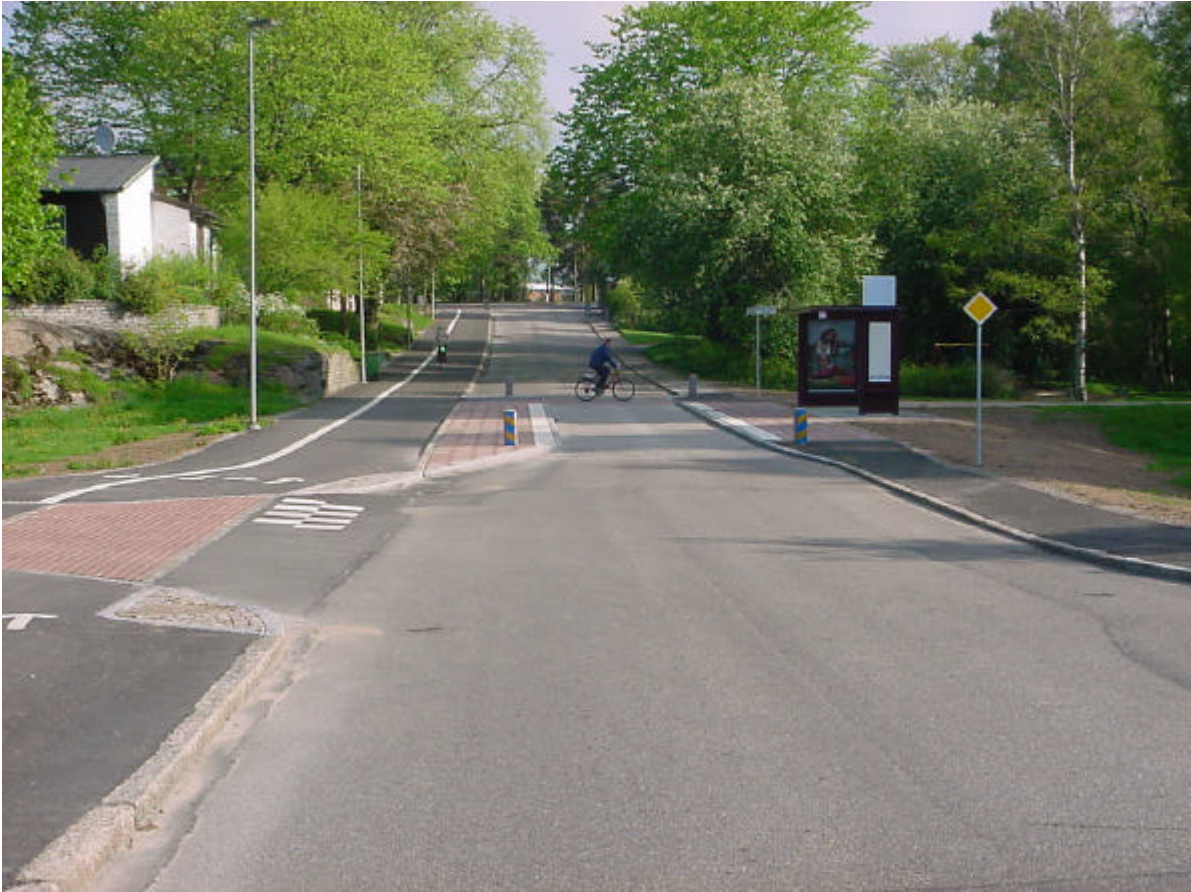
Figure 3 Example of a bus-stop from the en route to Vision Zero demonstration track
